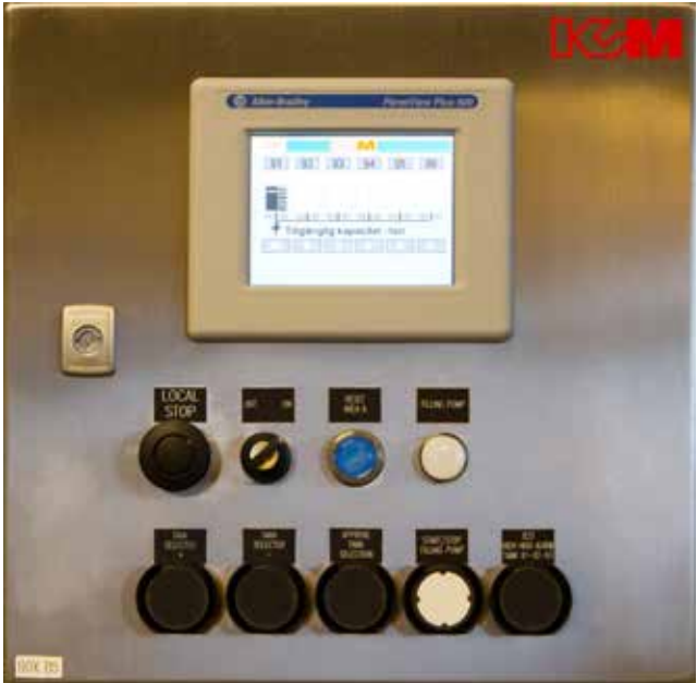
Filling pump control box with HMI display built into a stainless steel cabinet.
