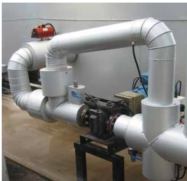
Dosing pump type HD6 with 3-way valve for local circulation.
