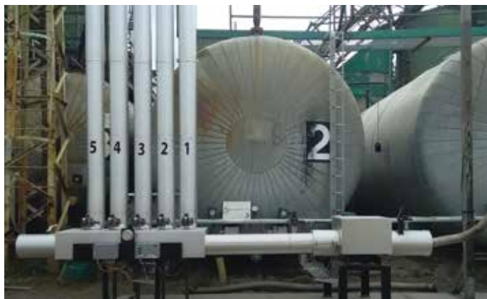
▲ Filling pump type HD8 and manifold with valves.
